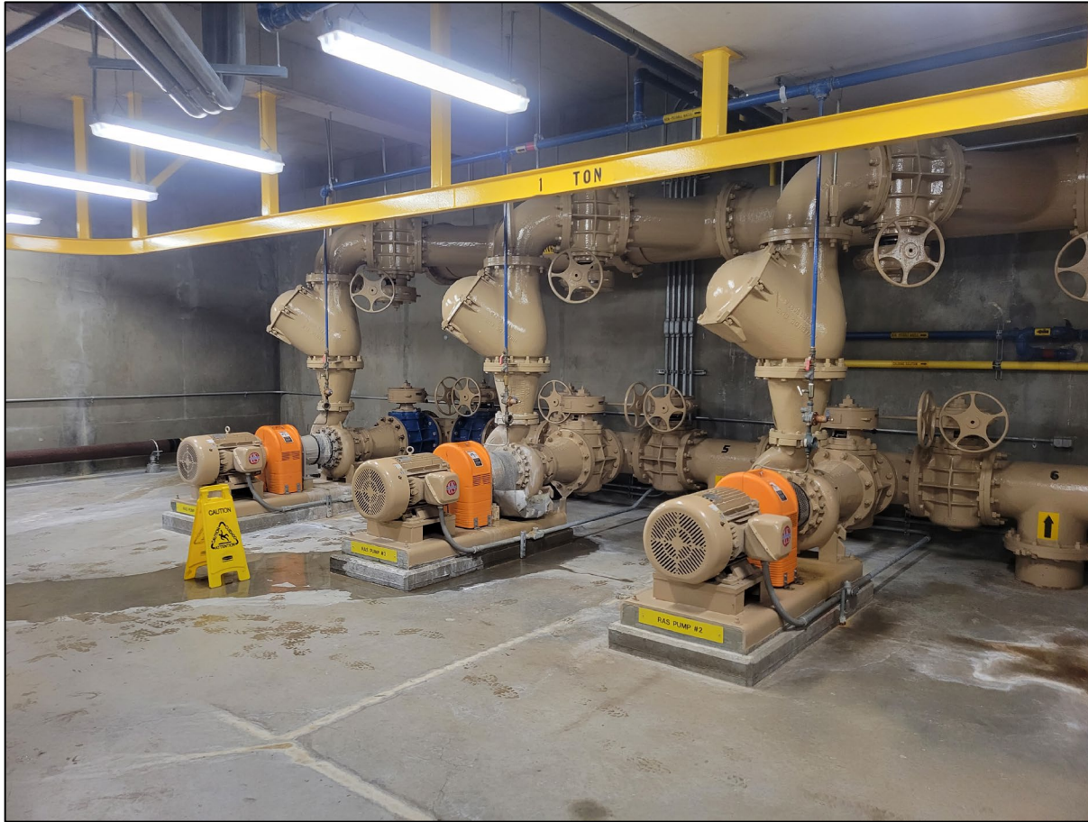
Leaking RAS valves at the treatment plant
