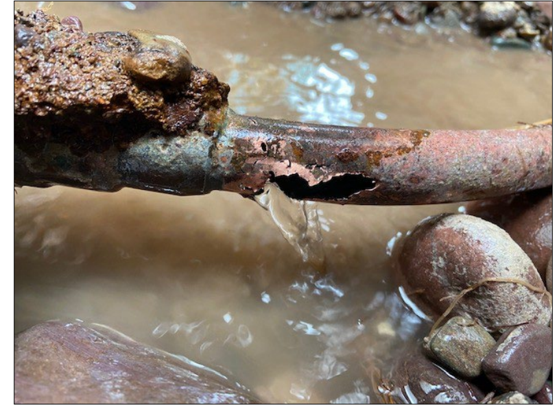
Examples of broken water service lines
