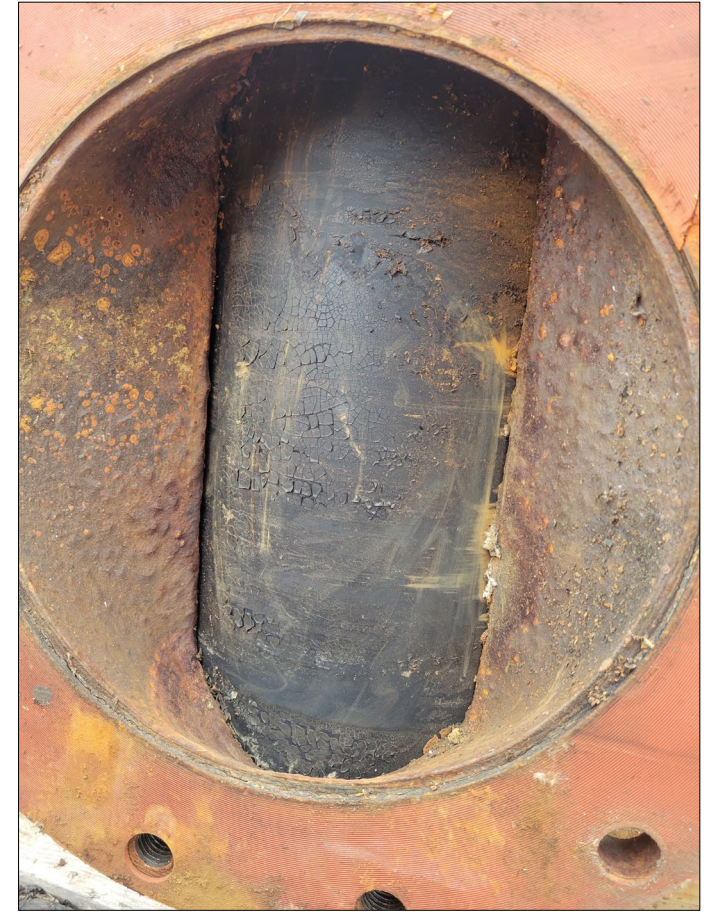
Rusty, corroded RAS valve
