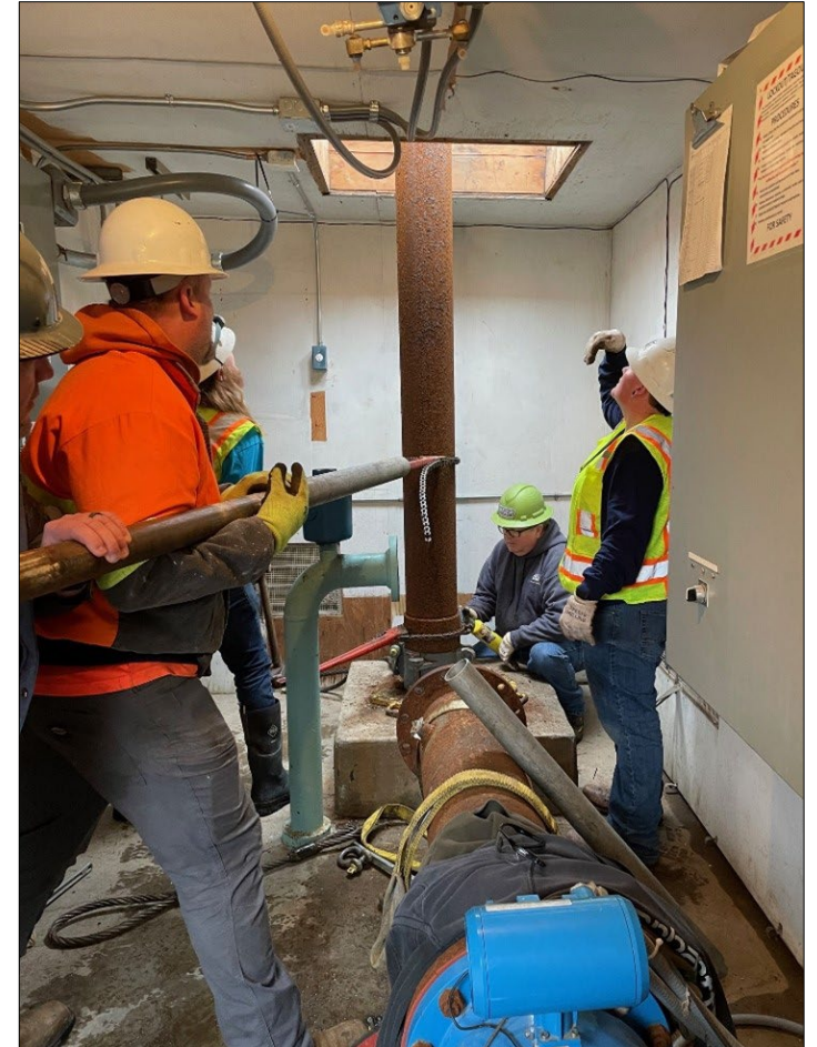
City Water Utility staff work with contractor to install new water pump
